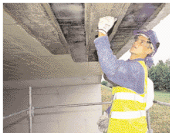
An ideal composite material for cold-bonded strengthening of concrete, steel or timber structures: TFC, which is used by Freyssinet for strengthening or conformity of all types of structures.
